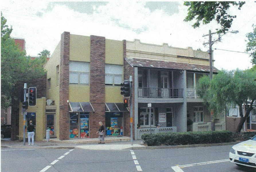
Figure 5 – Commercial development at 171 Blues Point, to the north of the sites Source: JBA
